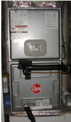
then runs out the drain line. There is always slime mold in your A/C Drain Pan. This is what causes a water backup in the unit. The mold builds up and then finally stops up the drain line. The drain line (left) should be checked on a
